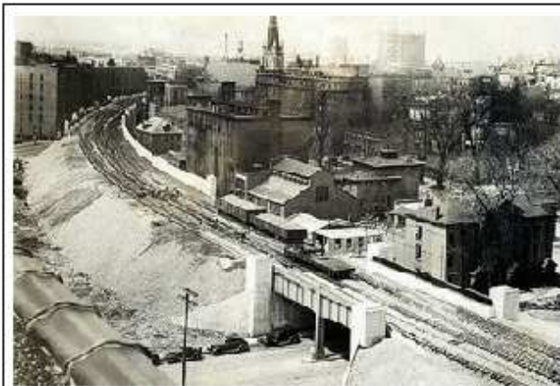
Track laying on new embankment
