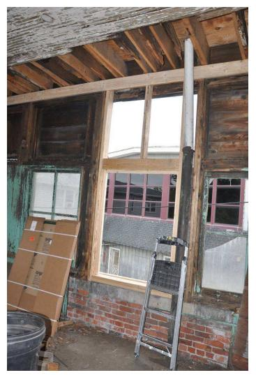
Left: Overview of reconstruction of a window frame and general view of tower upper level. Sadly, none of the original interlocking equipment remains, no levers, no control apparatus. Probably these were removed by the railroad in 1964 after the fire. October 25, 2018 *Jim Ball*
