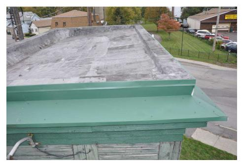
The roof is in good condition, the Chapter replaced the roof in 2004 and it remains in decent condition. Now with the addition of the aluminum capping around the roof edges, will go a long way towards making the structure more weather resistant. October 25, 2018 *Jim Ball*
